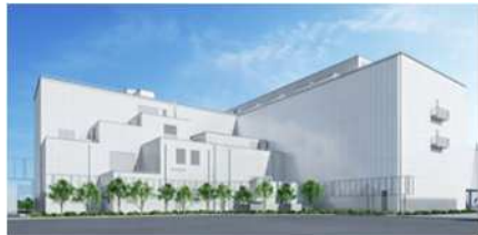
Main Factory Building No. 5
